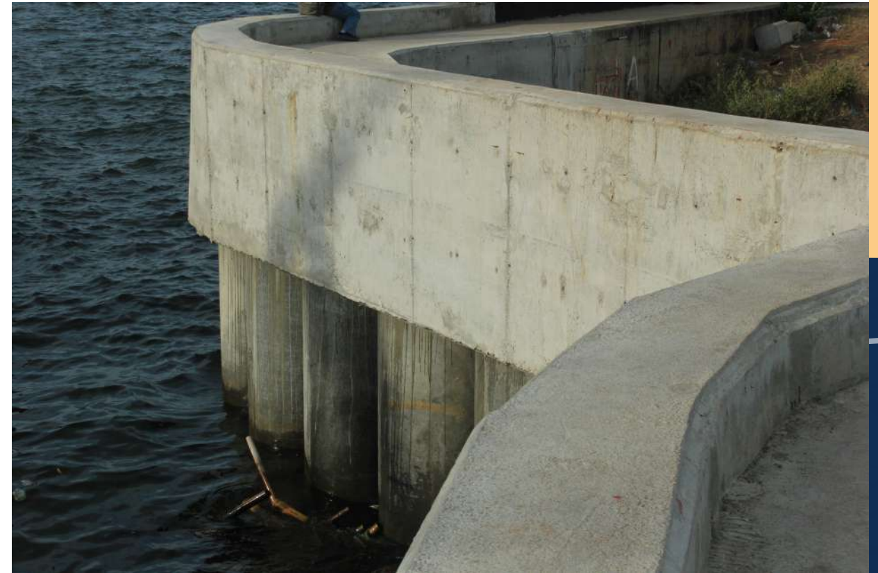
Tanggul Besar, 2022 The Giant Sea Embankment, 2022
